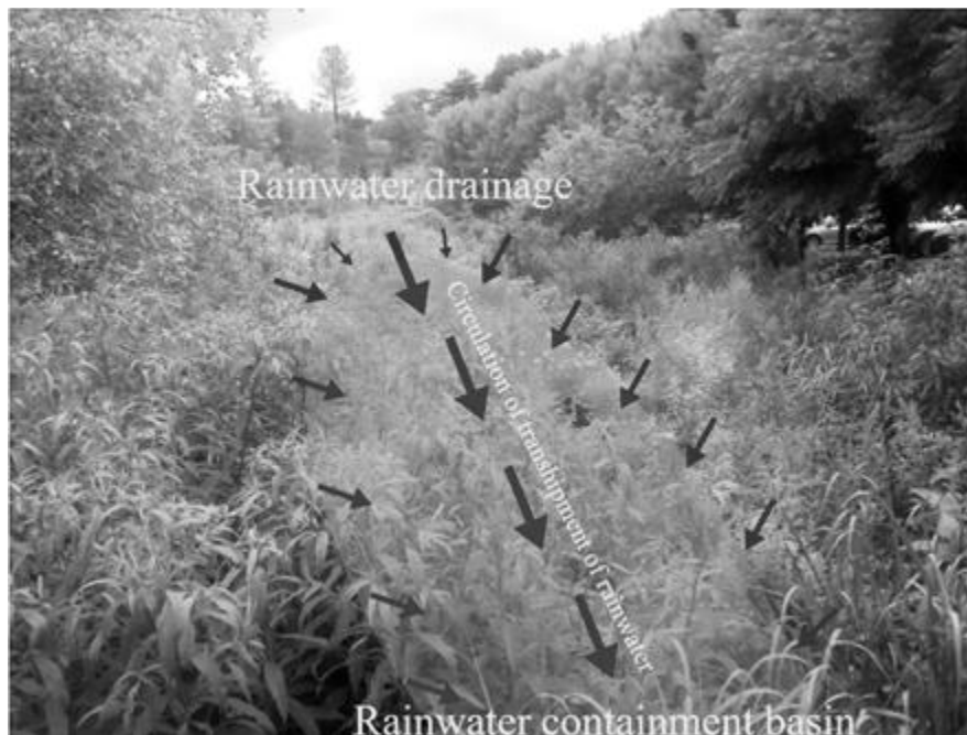
Figure 9 - Gardens integrated to the drainage system.
