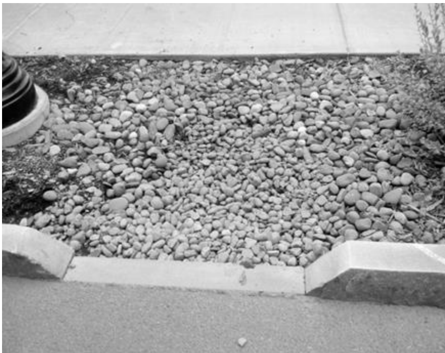
Figure 8 - Drainage at the site.
